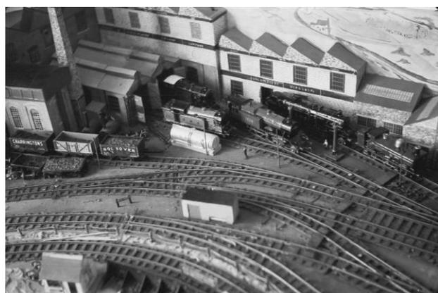
The track was a simple job, the centre rail just being pulled out and the eyelet chairs pressed down flush with the sleepers. The opportunity was taken to paint the running rail sides and sleeper tops in matt brown, giving a much more realistic appearance.
