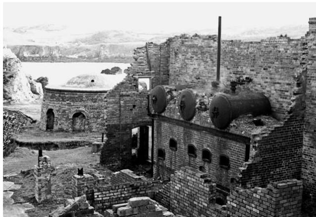
There are three circular brick-drying kilns (two of them retaining the original domed brick roof), interconnected by a large network of under floor flues leading to a tall chimneystack.....
