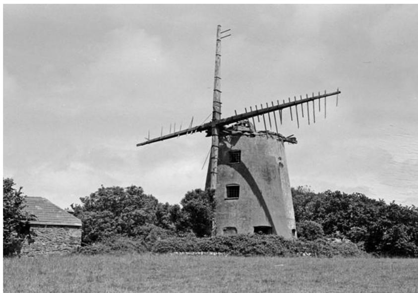
It was in a complete condition in 1934 when the Royal Commission of Ancient Monuments survey recorded it in great detail with a photograph and drawings. The tower is 30 ft 6 in high and has a diameter of 19 ft 6 in at the base; the span of the sails was 69 ft 6 in. On the top of the tower a timber curb carried an iron-gear rack upon which the cap was rotated to turn the sails into the wind, by means of an 8 ft diameter chain wheel.
