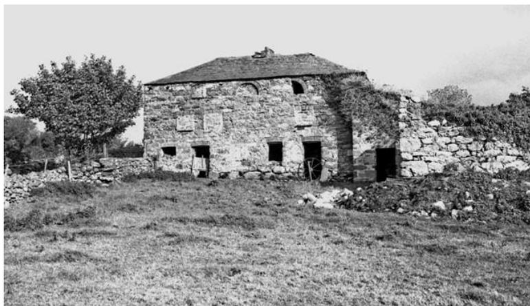
Nearby Felin Forgan, another corn mill (480567) disused for twenty years, retains its 18 ft diameter waterwheel which the owner intends to restore. The site used to be higher up the hill, and the story goes that the river changed course one night during a storm. The mill was carried down and rebuilt stone by stone by one Mr. Morgan, hence the name “Morgan’s Mill”.
