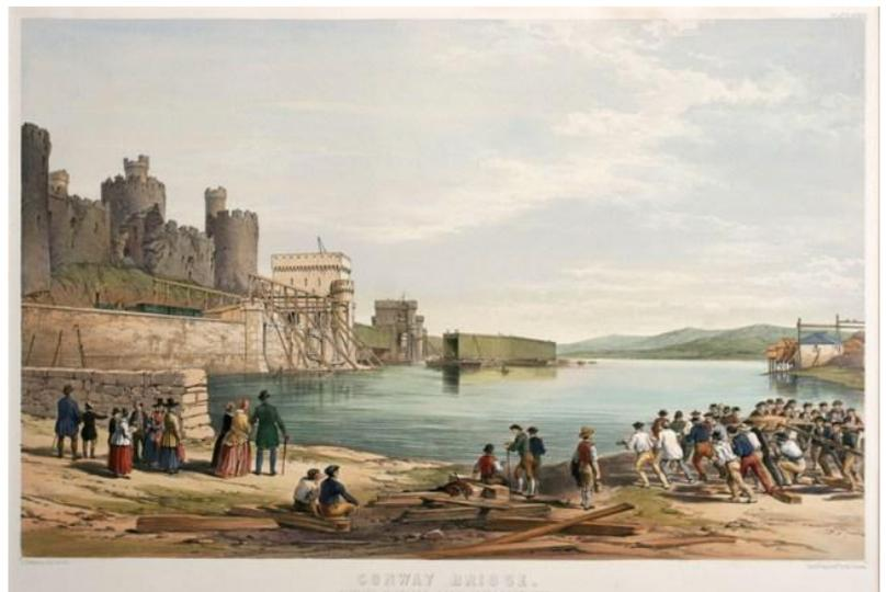
At Conwy, the "Medieval" stone towers were presumably an attempt to appease those objecting to the intrusion of the railway into the environs of the Castle. These towers, of Mona marble, support the twin tubes carrying the railway lines, each 400 ft long and weighing 1300 tons. On the inland side of the
